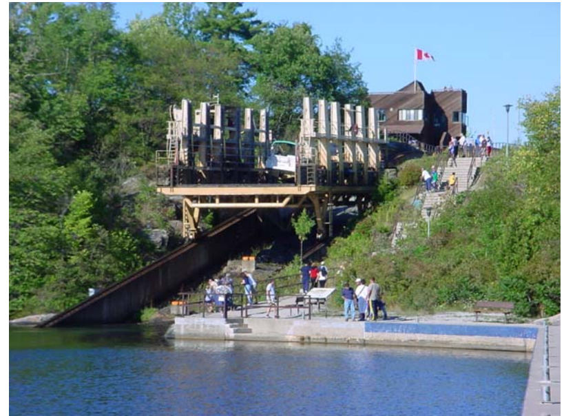
Marine Railway on the Trent Severn Waterway
