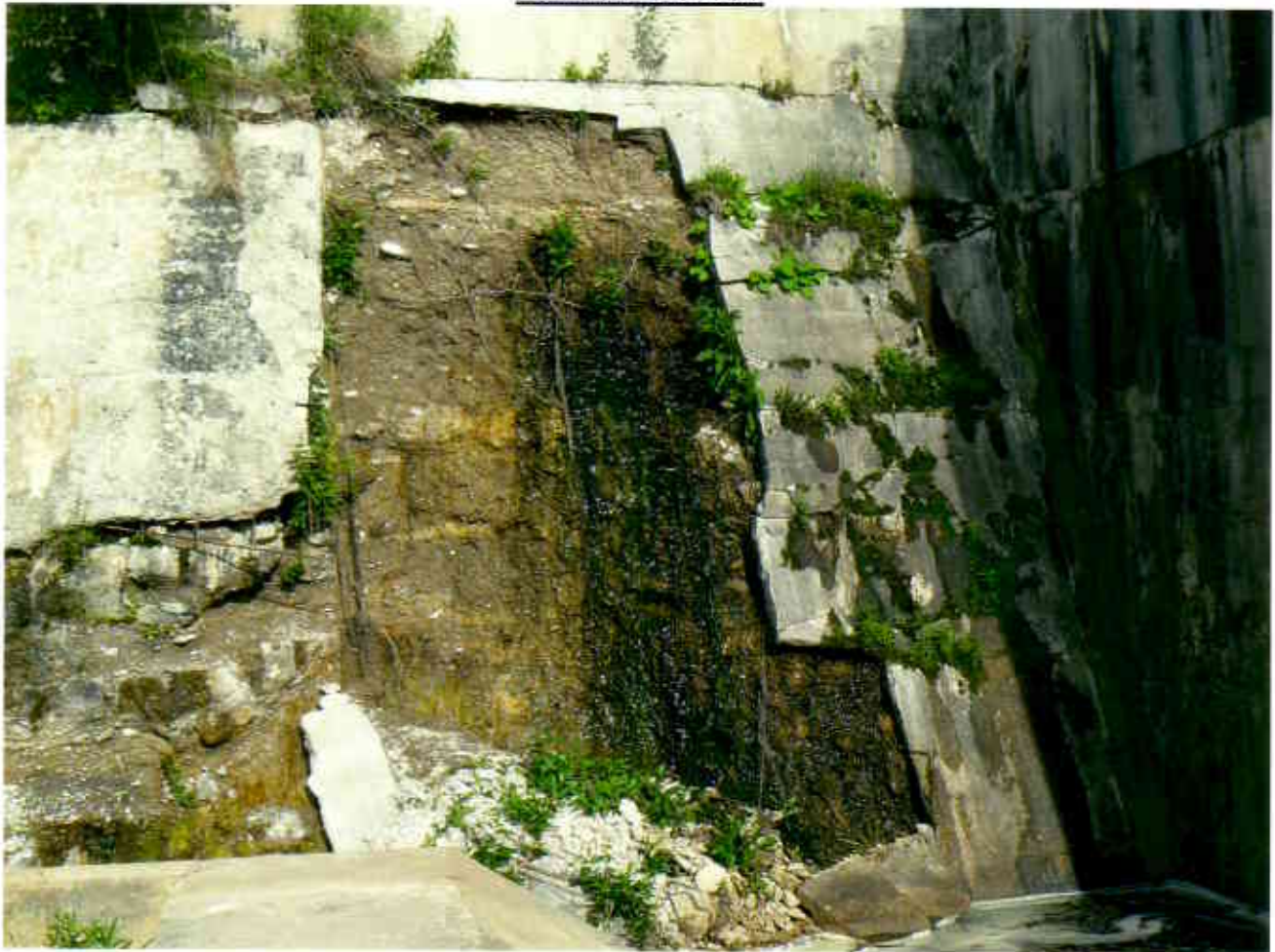
Dam at Lock 37
